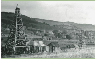
Drilling activity on the "flats" between Bolivar and Richburg
